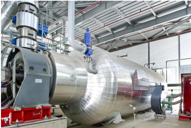
Surplus Geothermal Power ORC equipment identified
